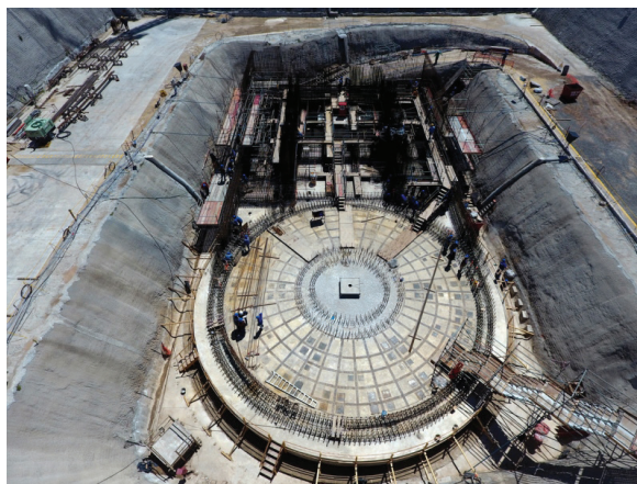
Figure 2: Construction works at the CAREM installation site. Credit: the CNEA.
