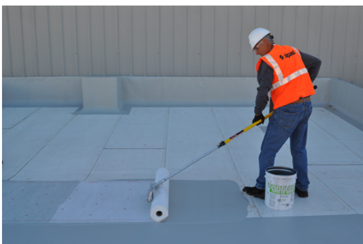
PMMA roof membrane systems are fully reinforced, layered applications consisting of one coat of primer (if required) and a waterproofing membrane comprised of two resin waterproofing coats and polyester fleece fabric.
