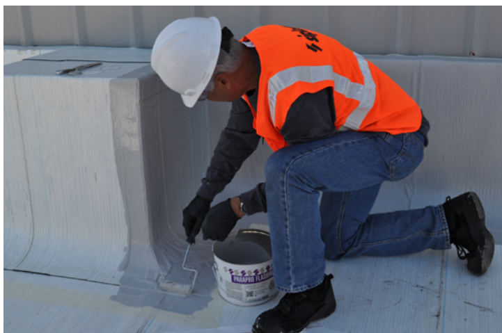
Fully reinforced, seamless PMMA flashing applications effectively address both standard and challenging details.
