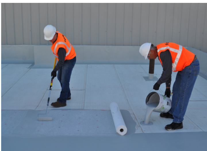
PMMA roof membrane systems are fully reinforced, layered applications consisting of one coat of primer (if required) and a waterproofing membrane comprised of two resin waterproofing coats and polyester fleece fabric.
